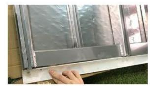
Install the Bar holder brackets at the top of the panels -this may require adjusting the PVC profile
